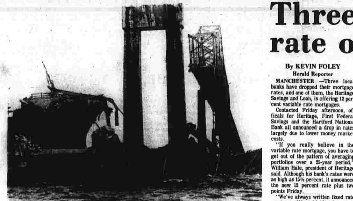
The 606-foot freighter Summit Venture sits off the western side of the toppled Sunshine Skyway bridge in St. Petersburg, Fla., with a portion of the fallen span astride its bow. Thirty one persons are feared dead when a Greyhound bus and several autos plunged into Tampa Bay. (UPI photo).
