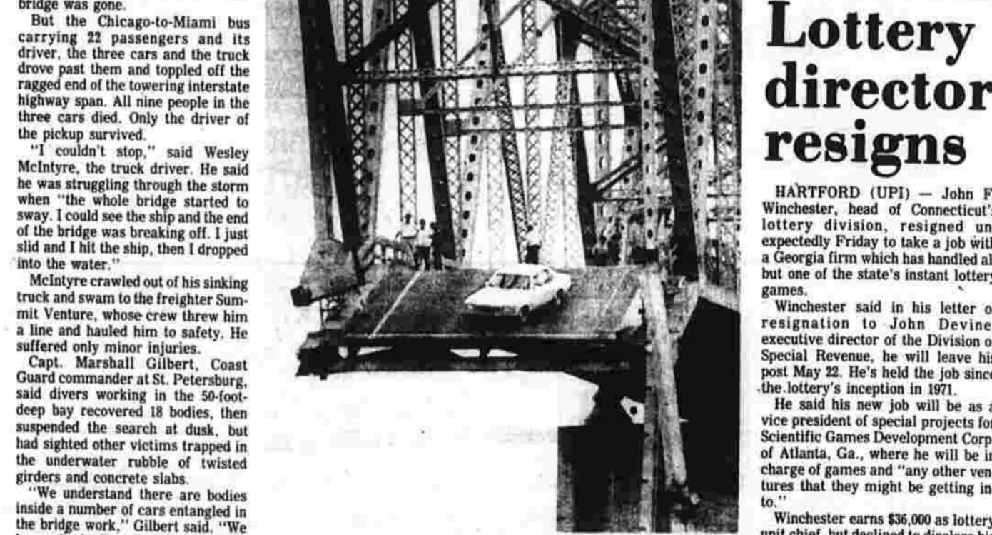
A car sits at the edge of the west span of the Sunshine Skyway bridge after the 606 foot phosphate freighter Summit Venture struck the bridge Friday during a storm knocking down approximately 900 feet of the bridge span. (UPI photo).
